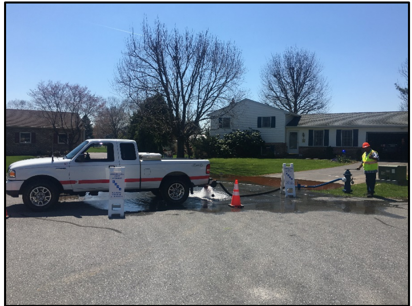
Figure: Flushing of Hydrant
